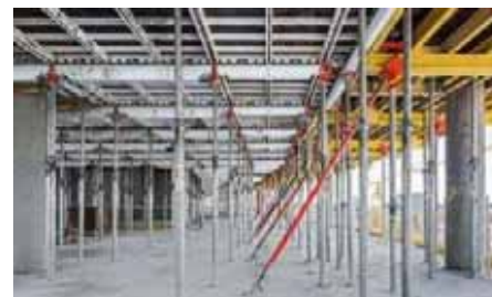
Aluminium formwork for B&C
