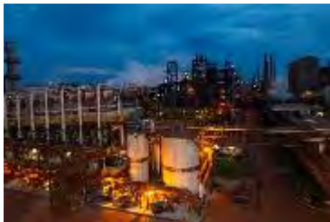
Start-up of new state-of-the-art dry disposal of bauxite residue using press filter
