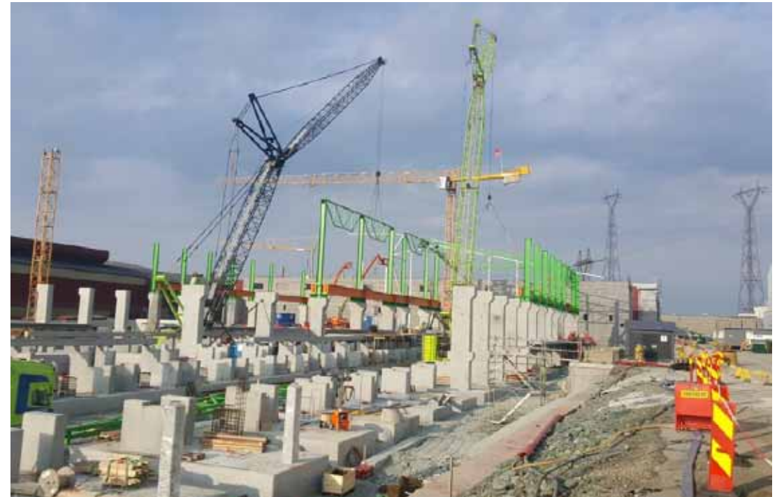
Potroom erection, incl. steel structure
