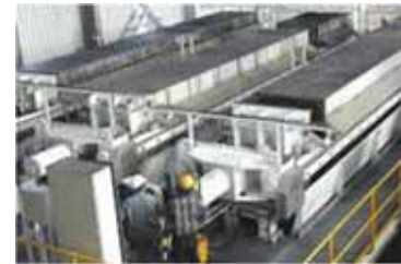
Commissioning of press filters at Alunorte
