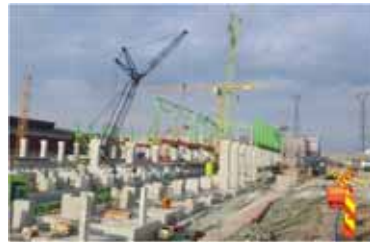
Karmøy Technology Pilot ~70% completed at year-end 2016
