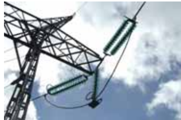
New power contracts to Neuss, Germany. Fully supplied until 2025
